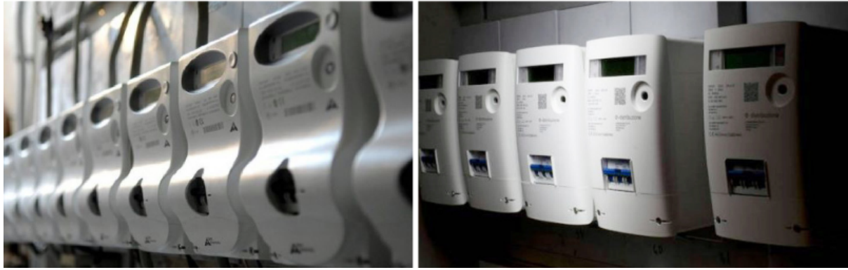
[Figure 1] On the left the first Enel Smart Meter, installed during 2000s in 32 million houses. On the right Open Meter 2.0, e-distribuzione smart meter, the second-generation meter with higher accuracy, ready for the smart home and equipped with interoperable communication protocol.
