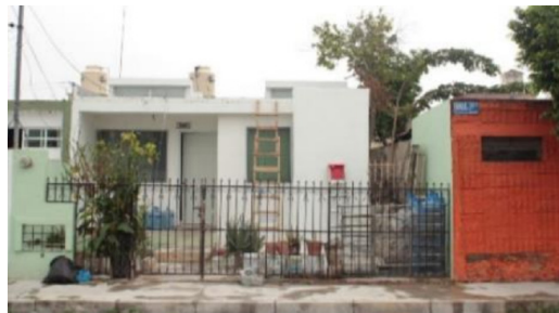
Image 6: Anahí Ramírez Ortíz Construction of ventilation for houses in Polígono 108
