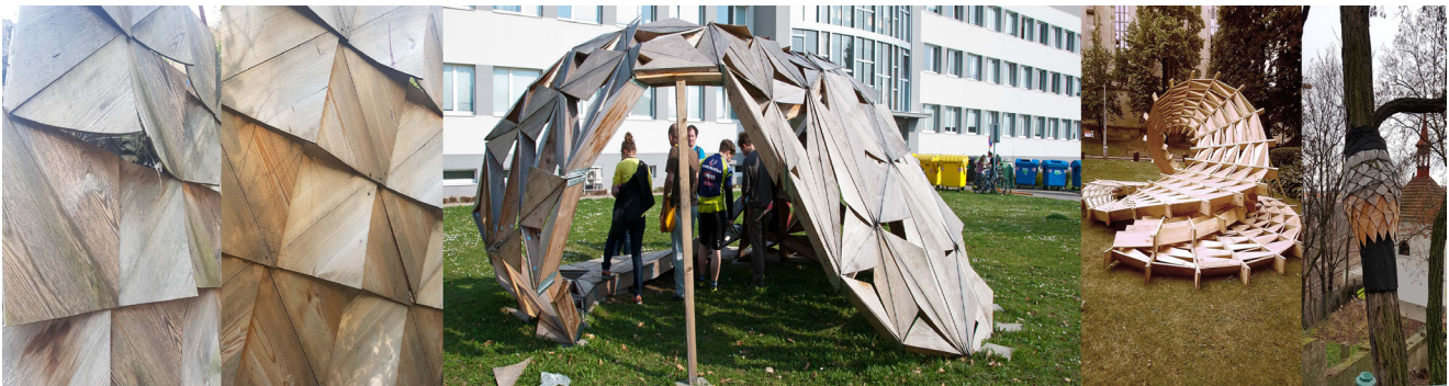
Figure 4: Different life stages after extensive weathering of wood responsive prototypes from left to right: a responsive screens Ray 2 after five years and a Ray 3 after three years, both inhabited by algae, lichen and blue stain fungus (the Ray 3 screen has washed out sugar by salt for preventing an interaction with decaying species); responsive pavilion pareSITE after one and half year of struggling with the interaction of torqued forces within the geometrical structure of Möbius strip with weather extremes of two summers and one winter; a collapse of the LOOP responsive wooden pavilion after the gardener ignored the requirement of turning of the sprinklers that watered the sunny oriented half of it in arid season (the pavilion was afterwards rebuilt at different location) ; and a responsive insect hotel TreeHugger CZ after one and half year fully co-performing with surrounding eco-system, being inhabited by both insects and algae. The prototypes were built within the framework of Collaborative Collective, Defio, s.r.o., Oximoron, Re.Code.Nature, ARCHWERK, Architectural Institute Prague, FA TUL, FLD CZU and CoLAND (photos: Davidová and Novotná 2014-2018)
